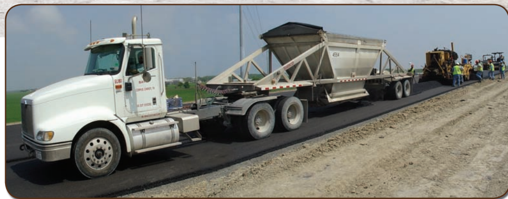
Above: The two-lane roads with concrete curbs being constructed at this time will one day be the frontage roads for a divided four-lane highway. Left: Bay Ltd. is underlaying these new lanes with 10 inches of Type A Grade 1 limestone base. The pavement consists of five inches of Type B asphalt overlay with two inches of Type C asphalt.
