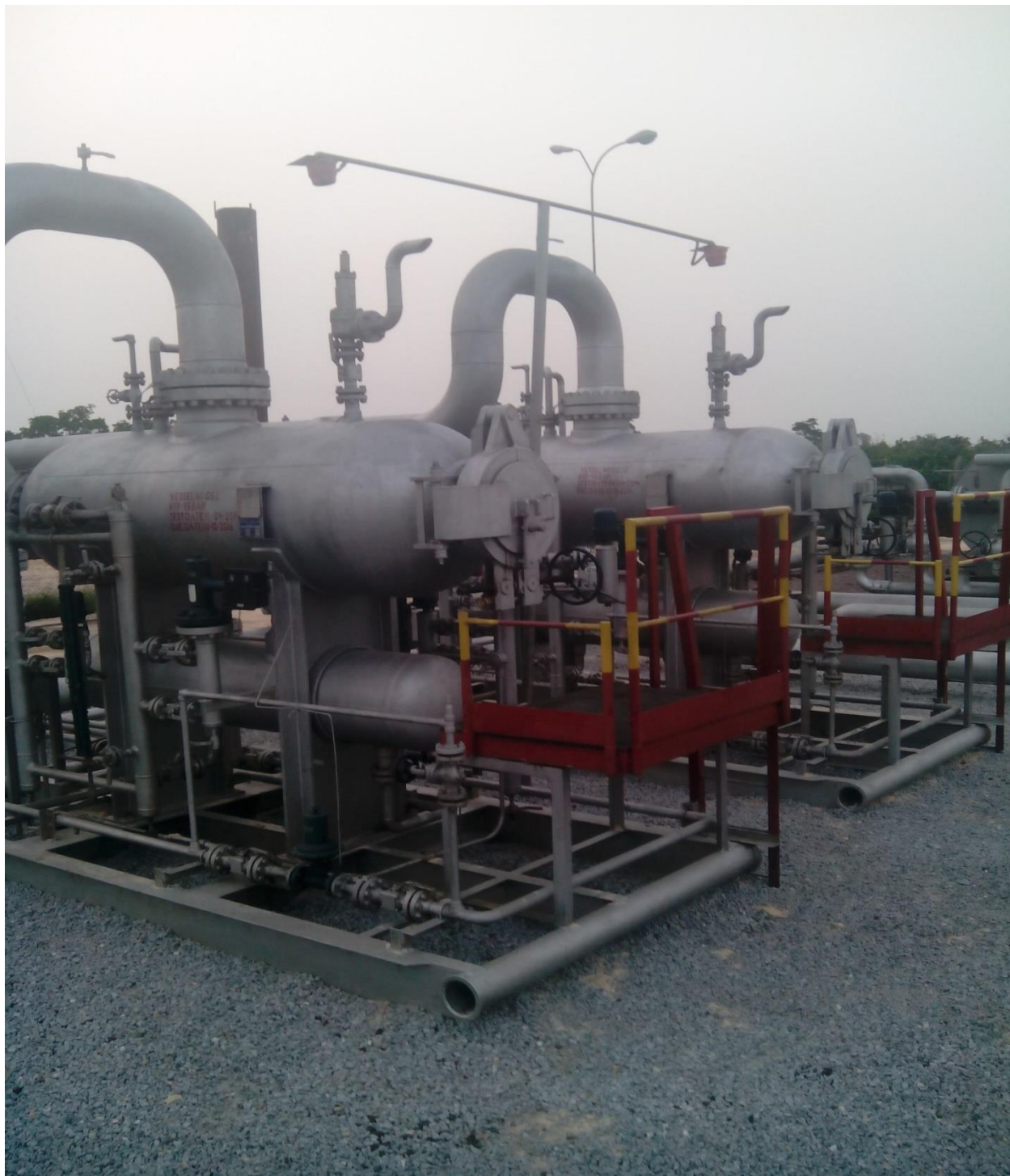
Figure 8: Gas Scrubbing Skid GS1 and GS2
