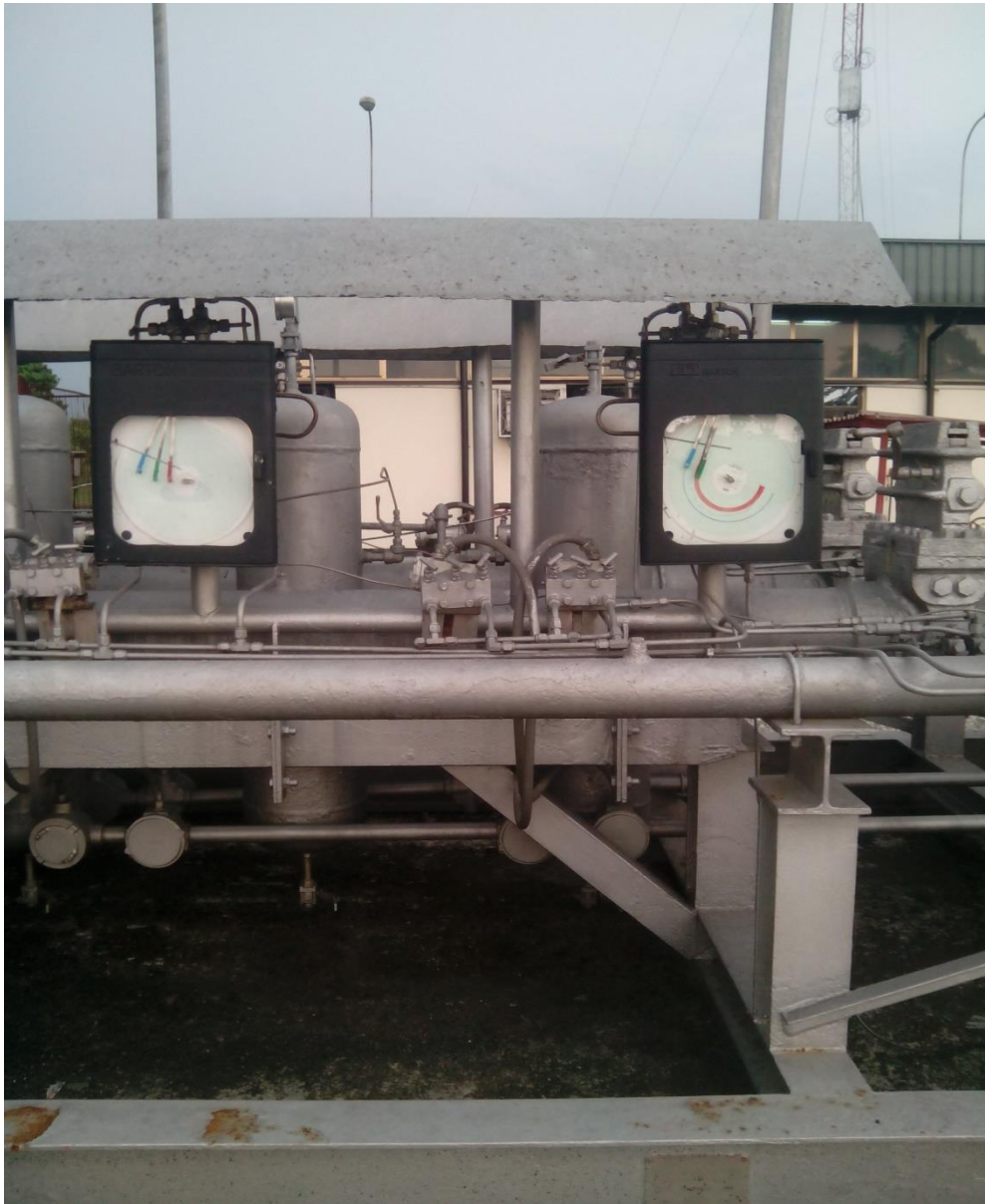
Figure 11: The Gas Metering Skid.
