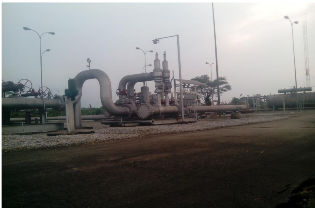
Figure 14: The Pressure Safety Safety Skid
