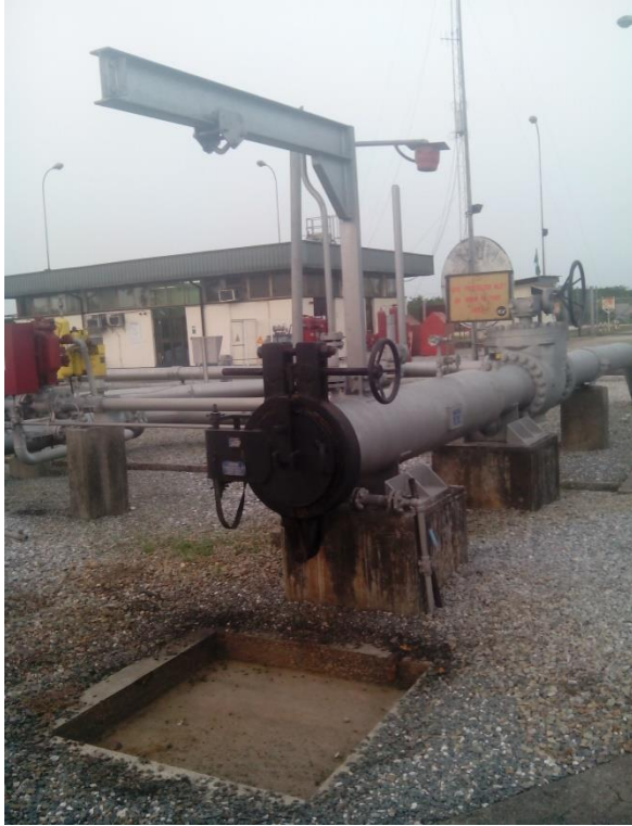
Figure 7: The Scraper Receiving Trap.
