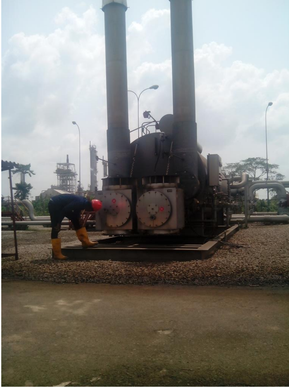
Figure 9: Indirect Bath Heater.
