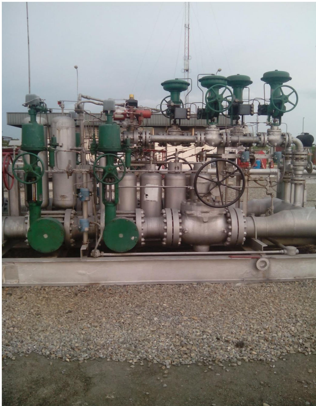
Figure 10: Gas Pressure Reduction Skid.
