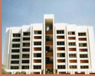
Residential Apartment for MUL Coop Housing Vapi, India Aug 1992 (M054)
