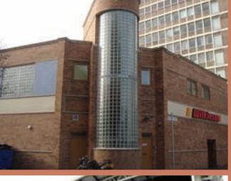
Wilkinson Store extension for Fara Estates Leicester, UK 1999 (W548)
