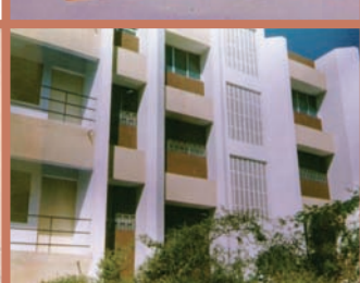
Residential Apartments for Gopal Housing Silvassa, India Sep 1994 (M094)
