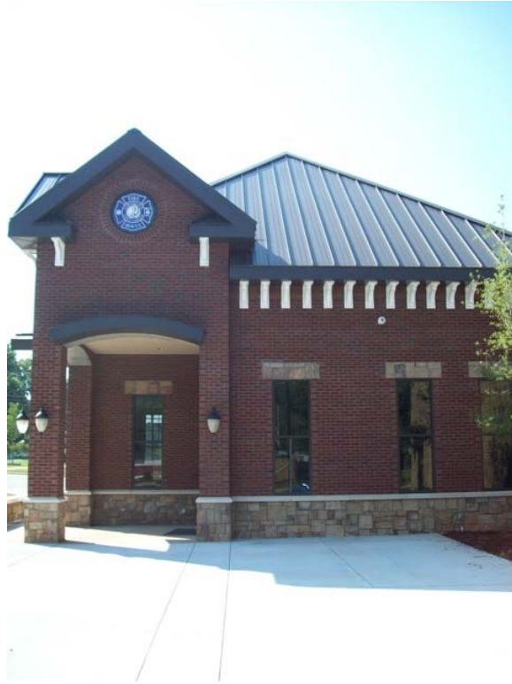
The Fire Department's Yagi is hidden behind the window at the top of the building to maintain aesthetics.
